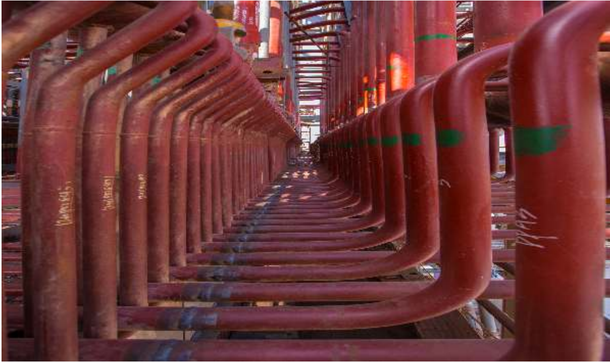
Welding of small-diameter pipeline of the boiler
