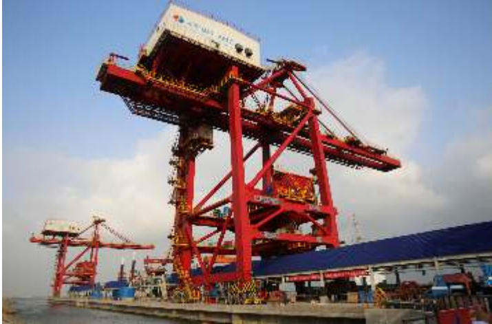
Complete view of in-house “Coal Unloading Jetty”
