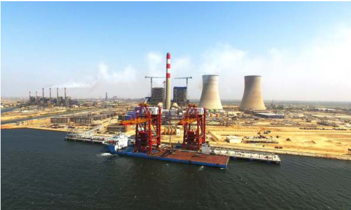
Whole view of “1,320 MW Port Qasim Coal-fired Power Plant”, 2017 (Under Construction)
