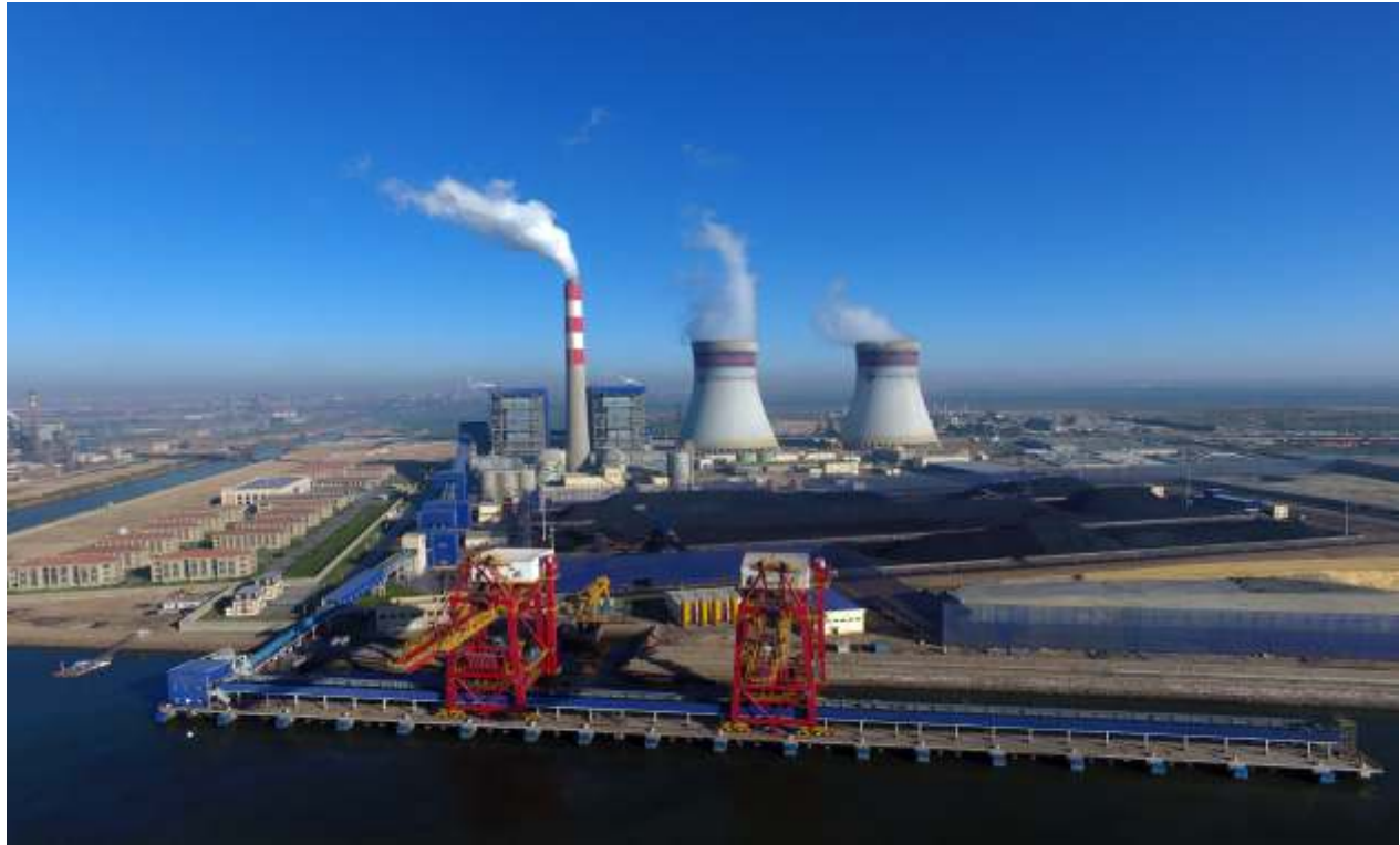
Complete view of “1,320 MW (Super Critical Technology) Port Qasim Coal-fired Power Plant
