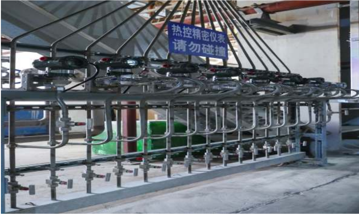
Installation of thermal control instruments
