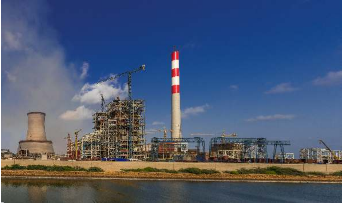
Whole view of “1,320 MW Port Qasim Coal-fired Power Plant”, 2018 (Under Construction)
