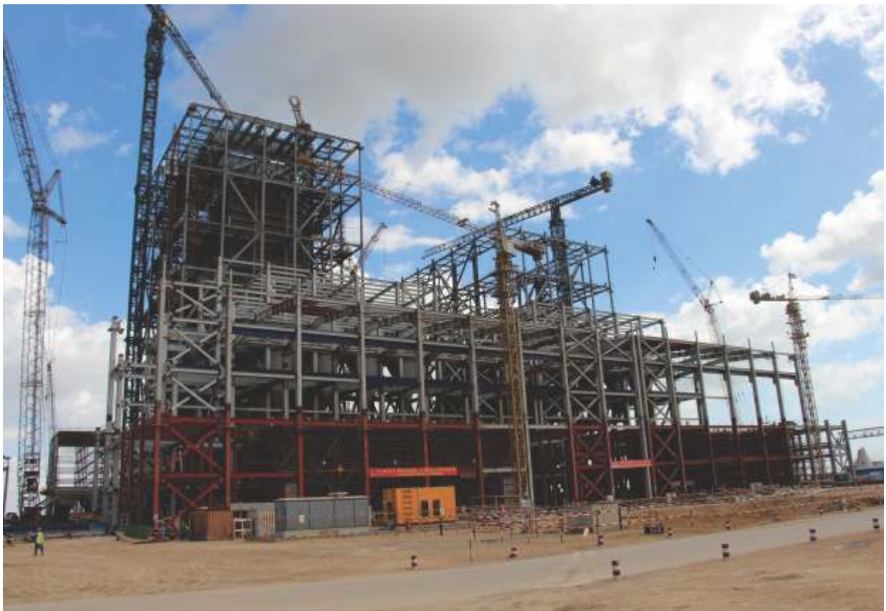
Figure 1. 1,320 MW Port Qasim Coal-fired Power Plant under construction
